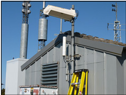
The slot antenna location - attached to the pole just to the left of the ladder below the large radomed yagi.
